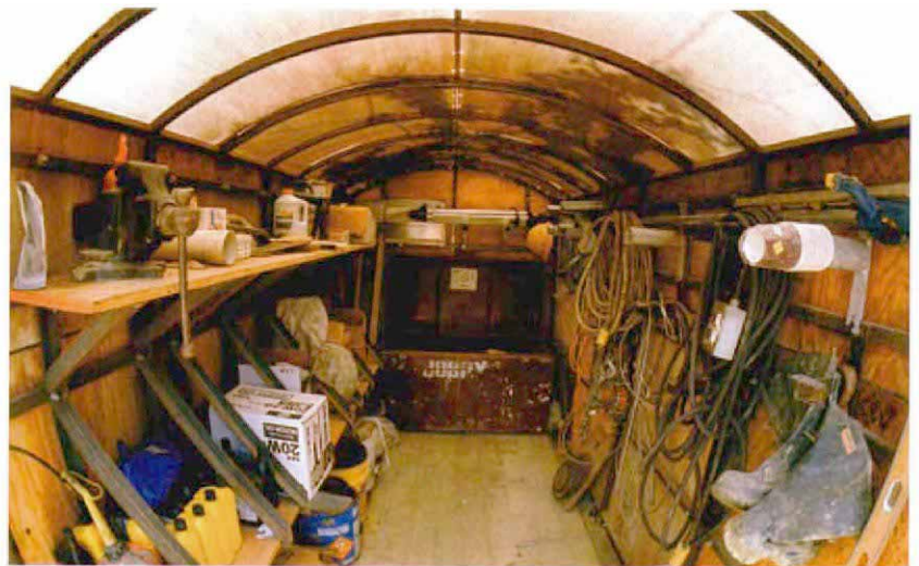
Translucent roof illuminates truck interior. To create a well-lighted storage area, Rockhill and crew covered the curved-steel roof frame with thin perforated sheet steel, followed by a layer of waterproof greenhouse fabric.
